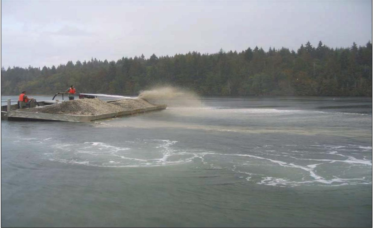
Figure 7. Graveling (frosting) over a clam bed
